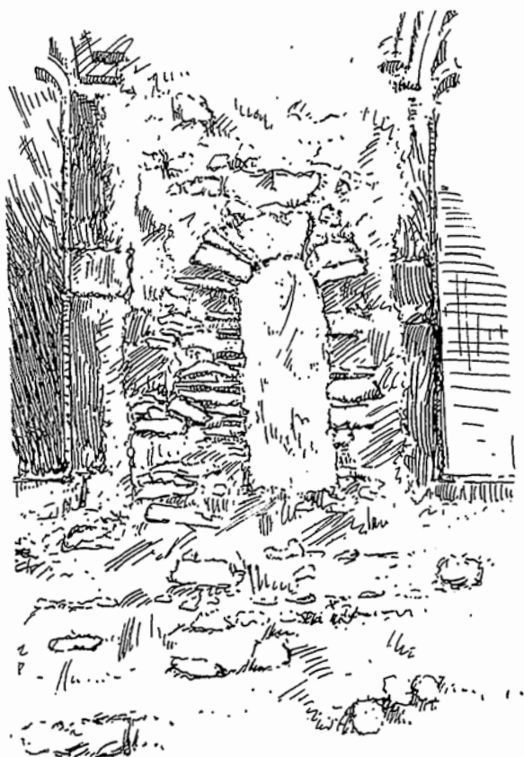
ALDINGTON CHURCH: BLOCKED WINDOW, (12TH CENTURY) IN EXTERIOR OF NORTH WALL OF CHANCEL.
