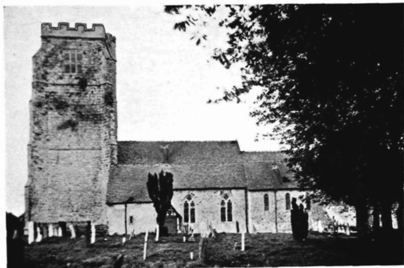
ALDINGTON CHURCH. From the South.
