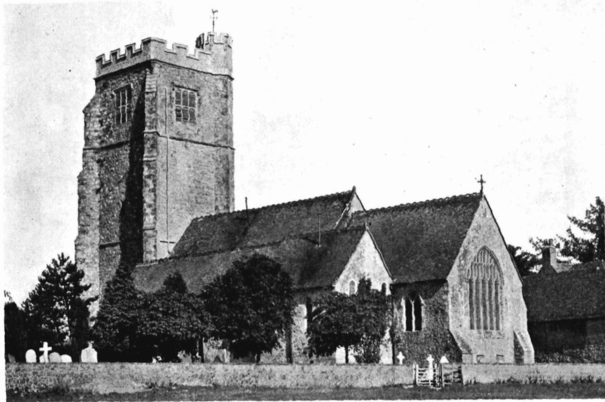
ALDINGTON CHURCH. From the South-East.
